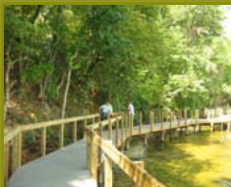
Park rangers attaching handrails to boardwalk
