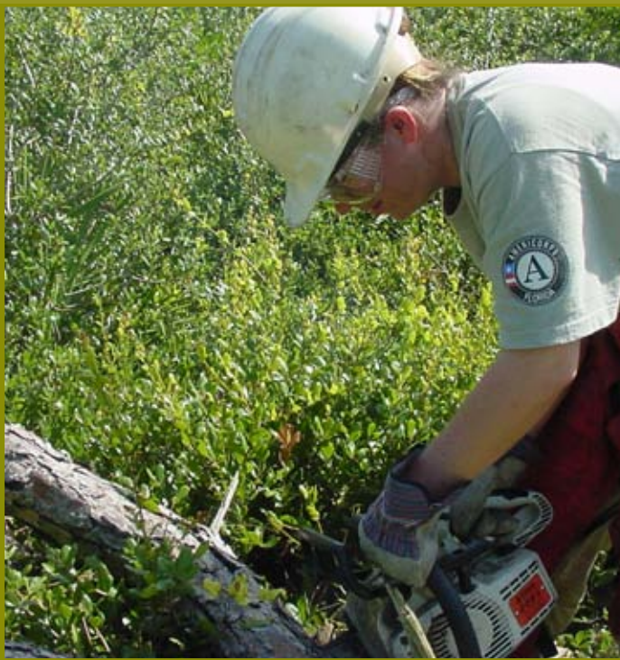
Jackie Crumbo clearing trails and roads with chainsaw after storm damage at Oscar Scherer
